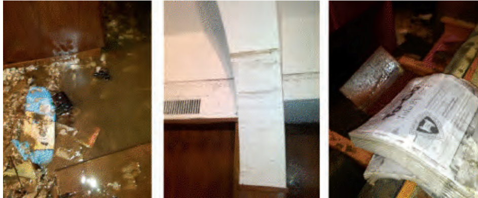
The destruction inside Congregation Ohab Tzedek in Belle Harbor
