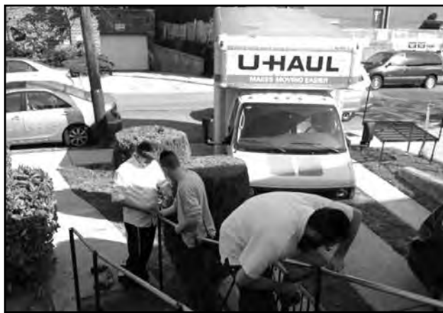
Wheelchair ramp being installed by volunteers
